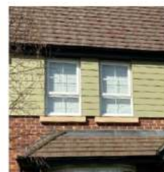
Timber panelling on upper storeys
