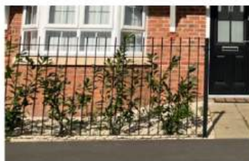
Black metal railings
