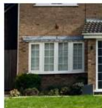
Bow windows with glazing bars
