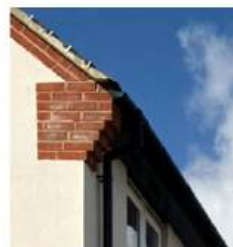
Stepped brickwork corbels
