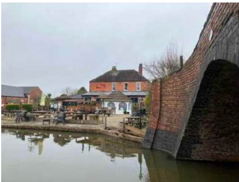
Photo of canal bridge and wharf, rear of Nadee's Restaurant
