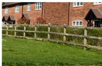
Rural timber paddock fencing
