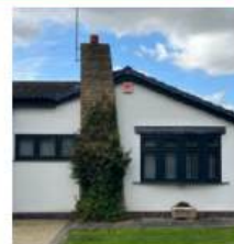
Feature stone chimney stacks
