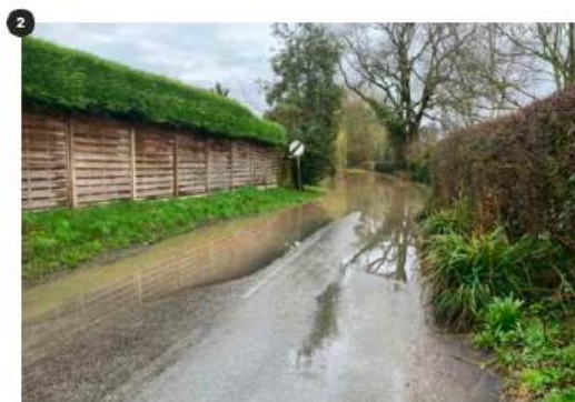
Figure 57: Flooding on Bakeacre Lane on 18th February 2024. An essential transport route providing key links to local schools.
