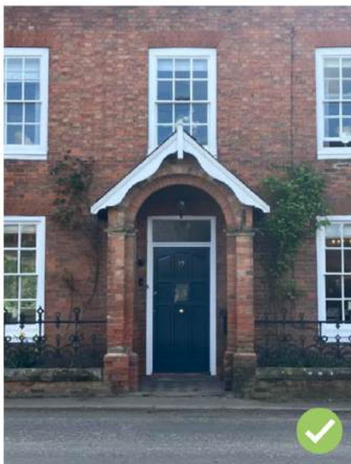
Figure 65: Containing many of the oldest buildings in the village, this area showcases character features such as sash windows and projecting porches.
