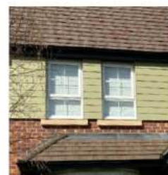
Timber panelling on upper storeys
