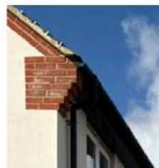
Stepped brickwork corbels
