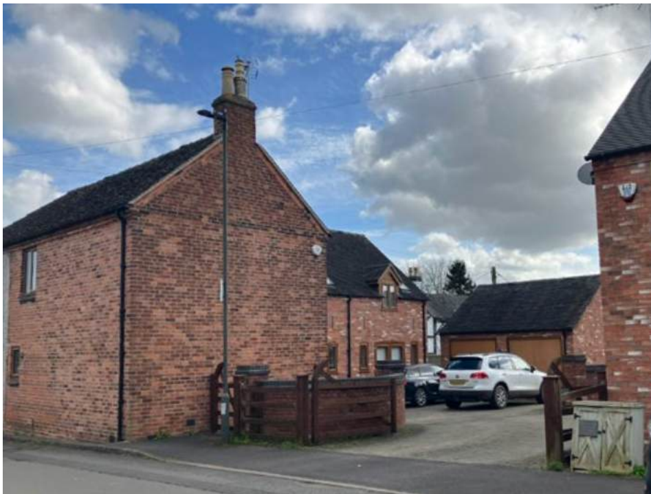
Photo of infill development well designed to harmonise with the scale, layout and materials of the traditional farm buildings with a cluster of buildings forming a courtyard.
