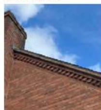
Dentil brick work along eaves
