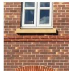
Brickwork banding
