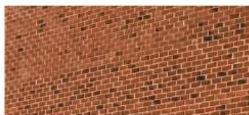
Red brick facades
