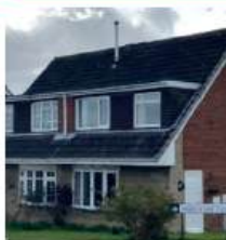
Large dormer windows
