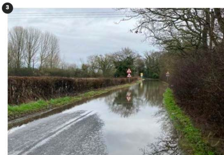
Figure 58: Flooding on Buckford Lane on 18th February 2024. Another essential transport route providing key links to local schools.
