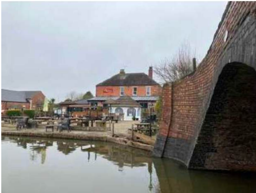
Photo of canal bridge and wharf, rear of Nadee's Restaurant
