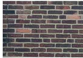
Red brick facades
