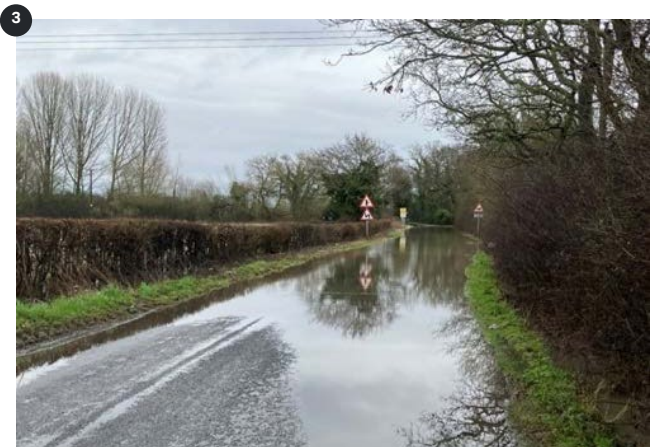
Figure 58: Flooding on Buckford Lane on 18th February 2024. Another essential transport route providing key links to local schools.
