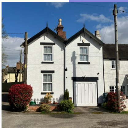
House + Cottage, nos 16 & 17, Lower Green
