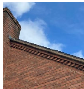
Dentil brick work along eaves
