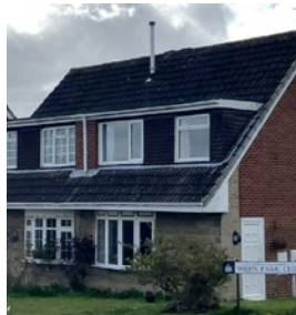
Large dormer windows
