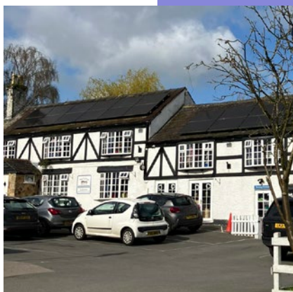
Old Forge Nursery Buildings
