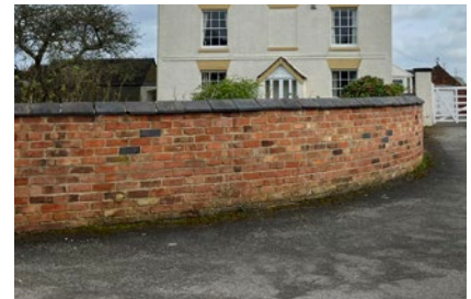
Medium rise brick walls with coping
