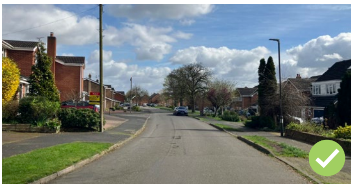
Figure 75: Key routes feature wide grass verges and generous footpaths, creating a pleasant environment for pedestrians.
