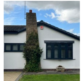
Feature stone chimney stacks
