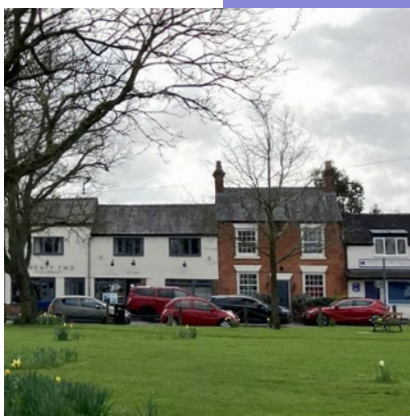
Group of 4 Houses, nos 22 to 24, The Green
