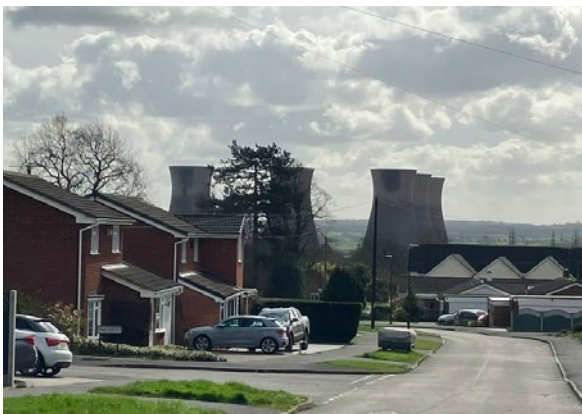
Figure 38: Former Willington Power Station cooling towers
