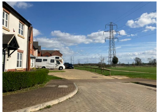
Figure 108: Development close to high voltage overhead lines at the edge of Highfields.
