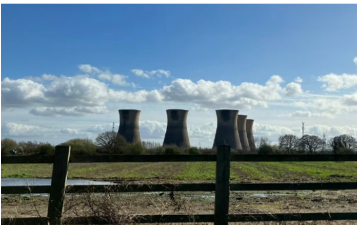
Figure 90: The cooling towers at the decommissioned Willington Power Station are a dominant skyline feature.
