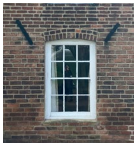
Paned sash window with curved or wedge lintels
